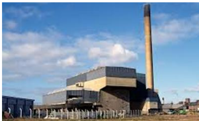
Figure 1 Eastcroft Incinerator in Nottingham
